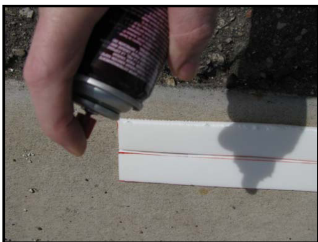
Figure 21: Apply spray adhesive to one side of each blade piece
